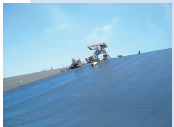
Zhanghewan Pumped-storage Power Station in China
