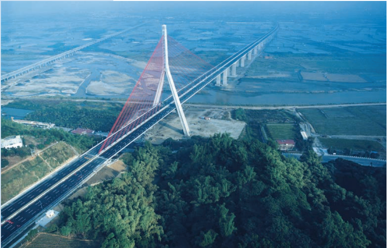
Cable-stayed bridge on the Second Highway in Taiwan (pavement on the bridge)
