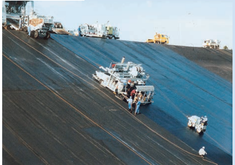
Kohyasan Dam (Asphalt facing)
