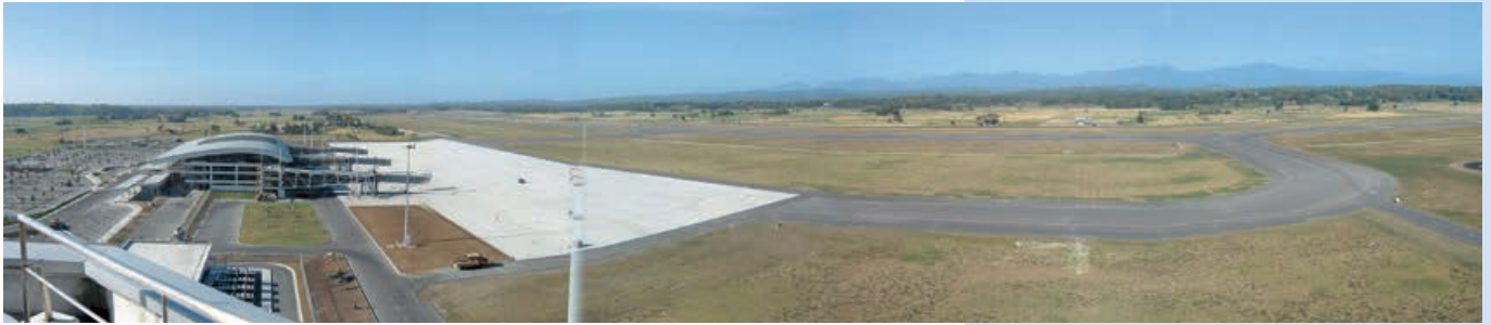
New Iloilo Airport in the Philippine
