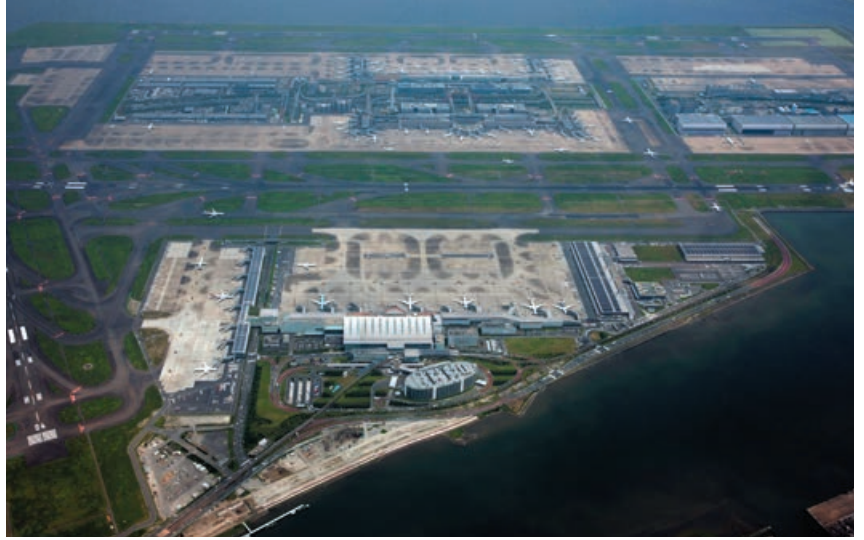
Tokyo International Airport (Pavement at Apron)
