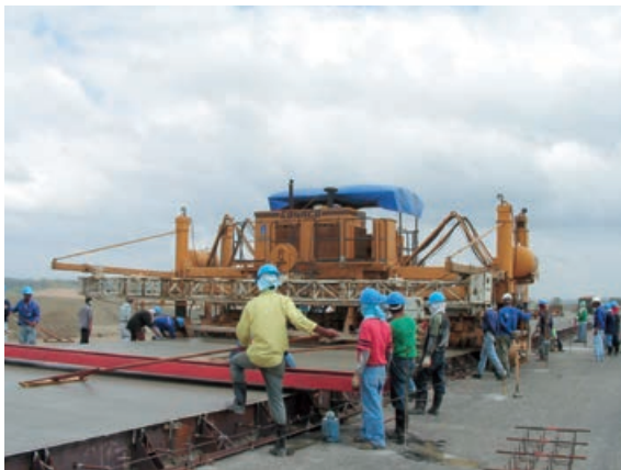
New Iloilo Airport in the Philippine
