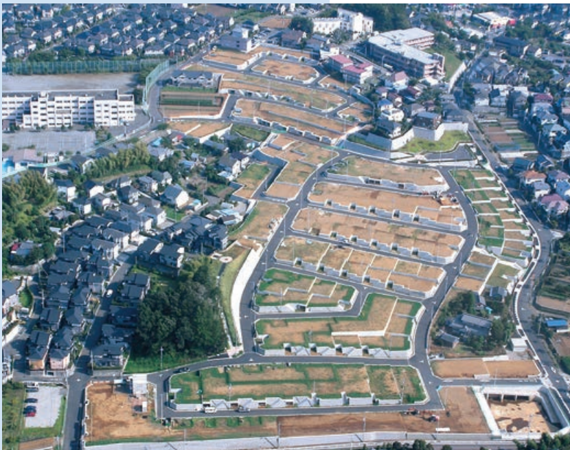
Kanai Central Land Readjustment Project
