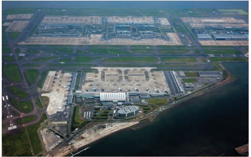
Tokyo International Airport (Pavement at Apron)
