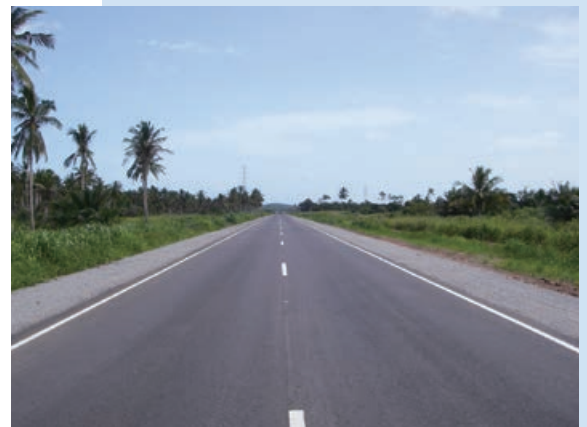
Arterial road in the Republic of Ghana
