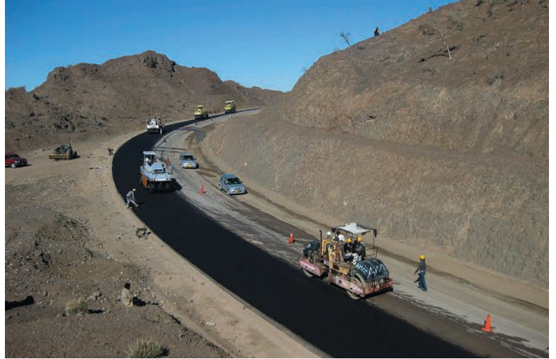
National Highway Construction PJ in Pakistan
