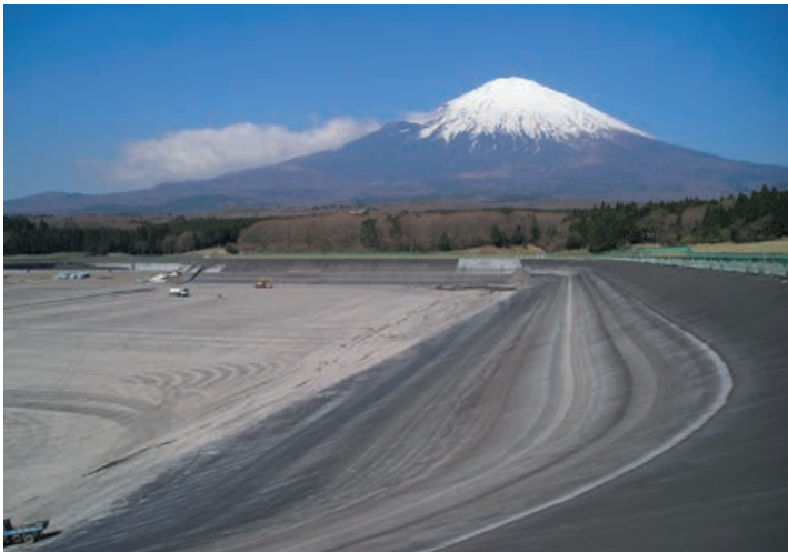
Prevention of Hazard in East Fuji Area (Asphalt facing)
