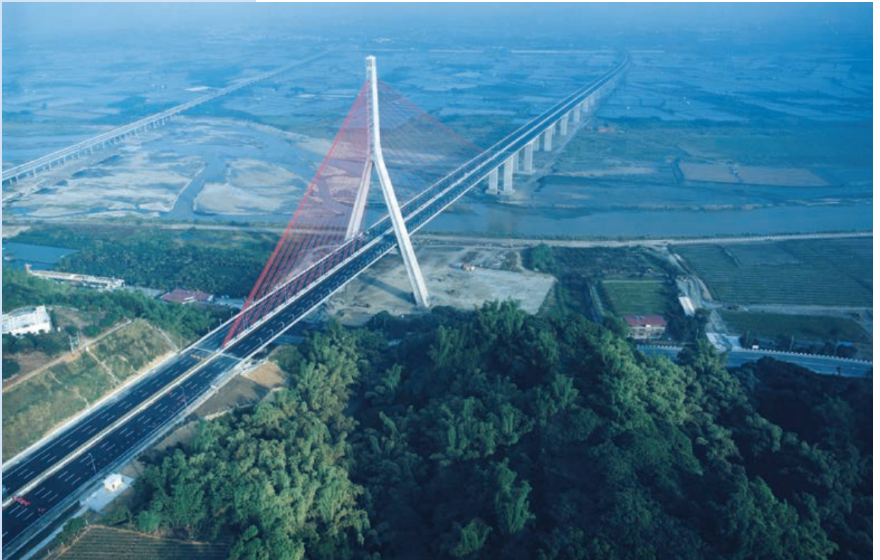
Cable-stayed bridge on the Second Highway in Taiwan (pavement on the bridge)
