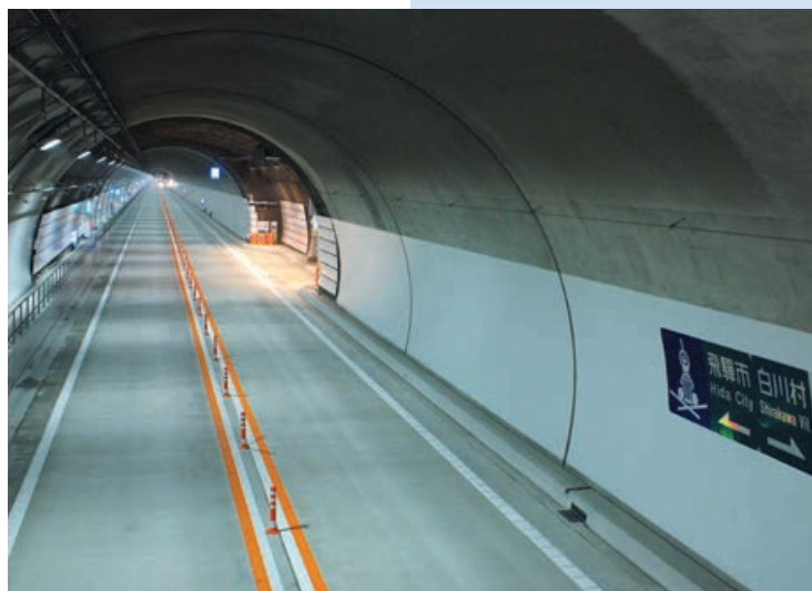
Hida Tunnel (cement concrete pavement)
